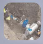
These drilling Machines are designed for under pressure drilling with a maximum working pressure of 16 bar. Suitable for drilling ND 65 to ND 200. Available in 3 different sizes. DN65 - 100; DN 100 - 150; DN 150 - 200.
